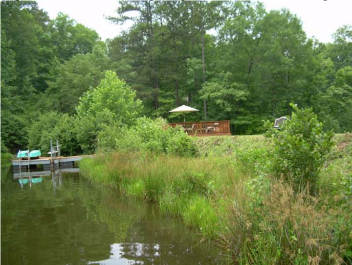
Figure 2. Observe emergent grass and short shrubs growing on the internal slope of dam.
